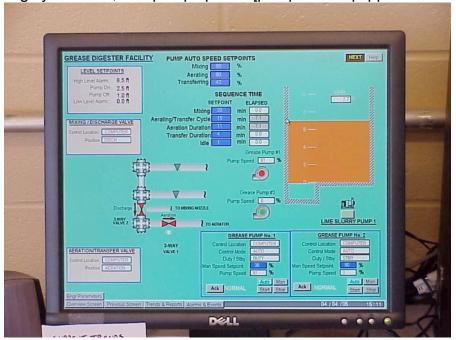
The operators control panel in the control room on an interactive computer shows all pumps and product feeds. From this panel the operator can monitor and actuate any of the equipment associated with the grease digester.
