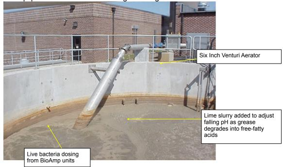
40,000 Grease digester tank shows the submerged discharge from the venturi aerator to maximize oxygen transfer. Small pipe protrusions are for adding lime slurry, and live bacteria from the incubator directly into the tank.
