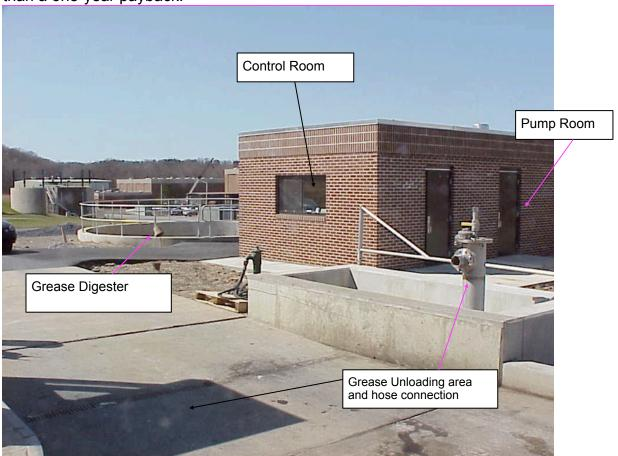
The grease hauler drives his truck up to the unloading station. The operator checks the gallonage in the truck for billing purposes and examines the grease to ensure it's not commingled with septage. [Current rate is \$85/1000 and will be raised at the end of the year]. The hauler connects the hose to the pipe stantion quick connect and begins off loading his grease.
