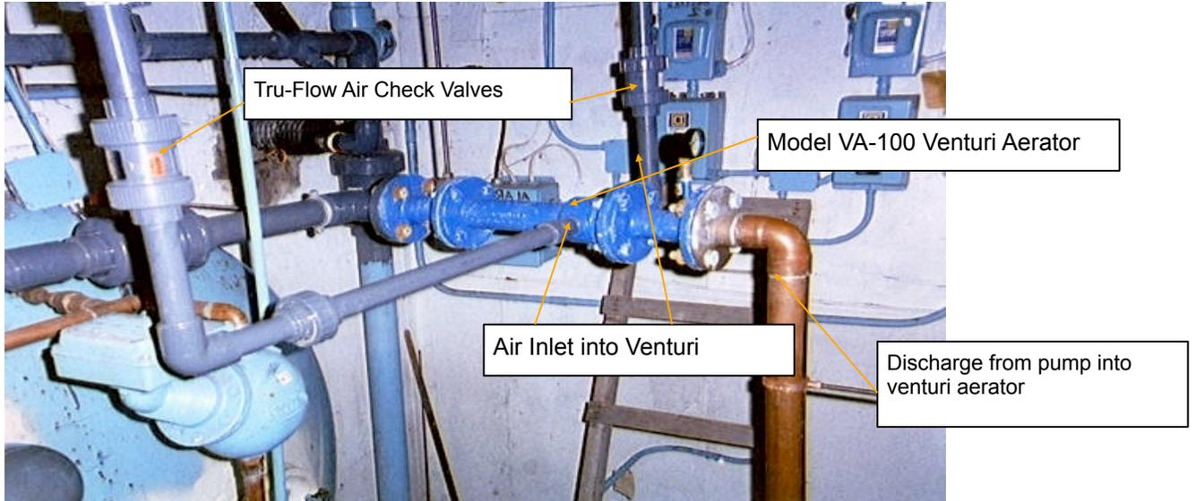
In the case at Pelham High School, PCE is stripped using the venturi aerator system to N/D (non-detect) levels making the water acceptable for drinking, cooking, showering and landscaping. Further, stripping carbon dioxide non-chemically adjusts pH from acidic to neutral levels. The addition of chemical alkalinity *is not required* for corrosion control. A side benefit of the venturi aeration process is the stripping of soluble radon gas to levels below 300 pCi.
