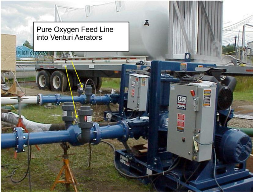
The two venturi units with the LOX feed are directly treating only ~3.2 million gallons of the 42 million gallon effluent but the kinetic energy of the subsurface discharge is allowing for additional mixing and equalization prior to the liquids entering the middle of the lagoon through a 300 ft long pipe. This ensures maximize utilization of the pure oxygen feed to ensure good economic return.
