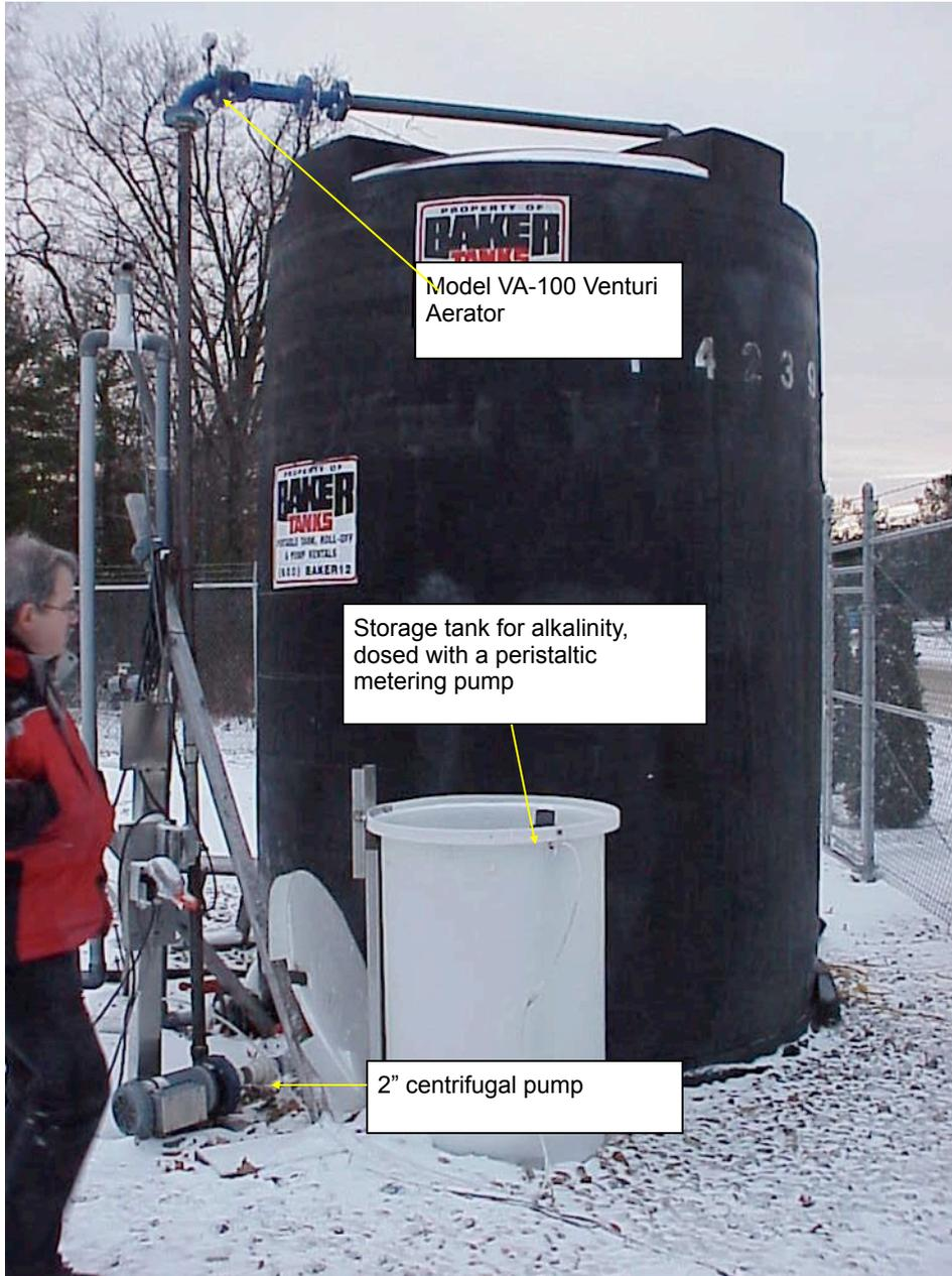
The entire treatment process time was two days from when the wastewater was pumped into the aeration tank until it reached a very large leaching field after the two trains of BioClere trickling filters and a Dynasand denitrification column. Residual
