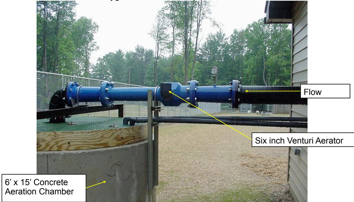
Using this venturi aerator configuration the Treasure Lake WWTP is able to maintain DO levels of  $>10.0$  mg/L in the cooler winter months when oxygen is more soluble in the colder water, while in the summer months they consistently exceed 7.0 mg/L when the air and water are warmer. This is in excess of their 6.0 NPDES permit and keeps them above their discharge permit requirement.
